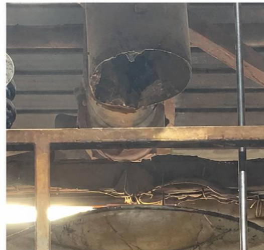
Leaking Floor Drain
